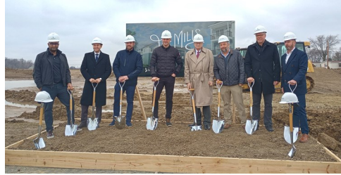
The Mills broke ground early in 2024 in Sidney. At completion, this project will offer 216 new apartments with a variety of amenities.
