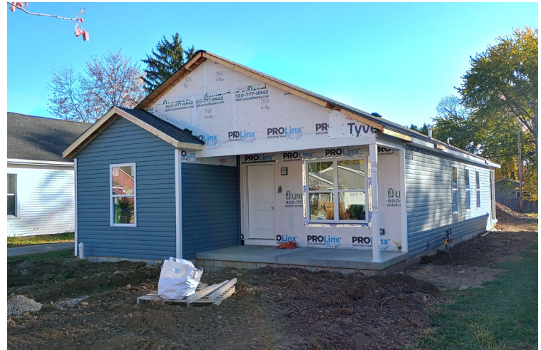
732 Broadway Ave, Sidney (Home is near completion)
