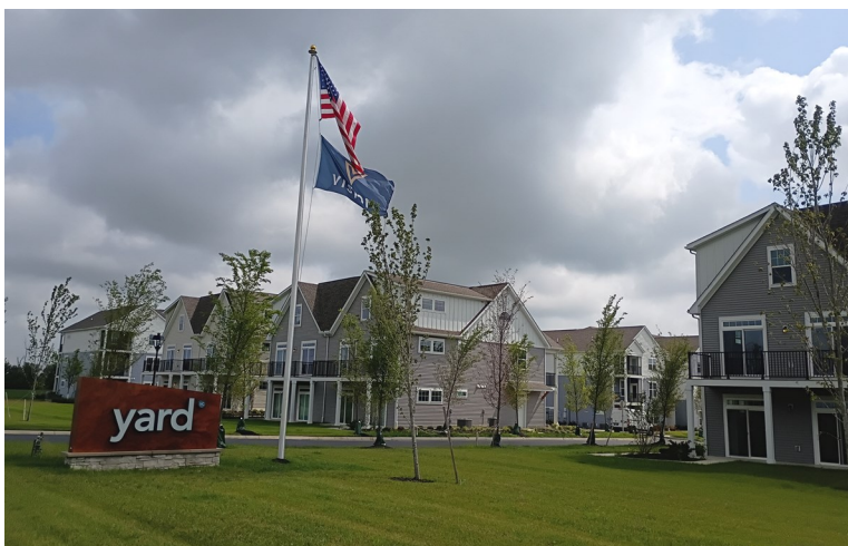
The VC Yard apartments at 1000 N. Kuther Road in Sidney is now leasing one, two and three bedroom apartments. A total of 220 units will be available at completion. Visit www.vcyard.visioncompanies.com for more information.
