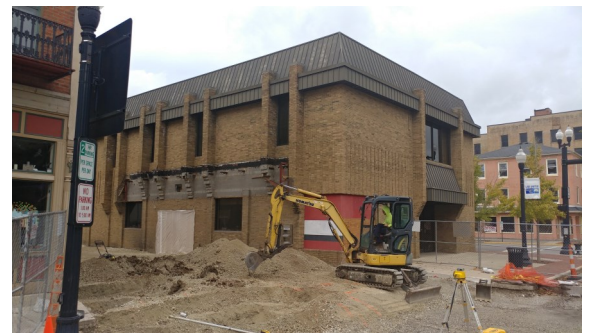
Work is underway at 101 S. Ohio Ave. in Sidney
