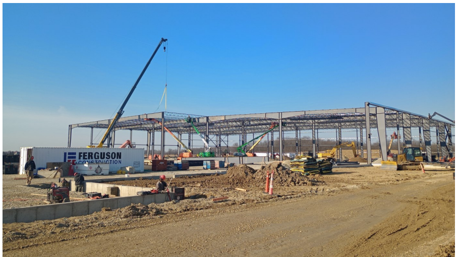
SEMCORP building #2 progresses on Millcreek Rd in Sidney
